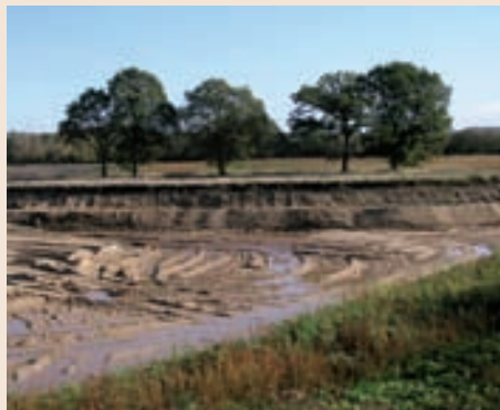
Landscaping to create the lake terraces.
